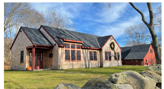
SKLT Offices at the Woodcock Campus at Weeden Farm
